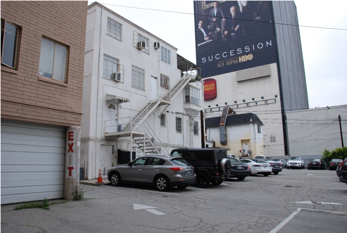
Figure 3a South Side of Project Site looking East
