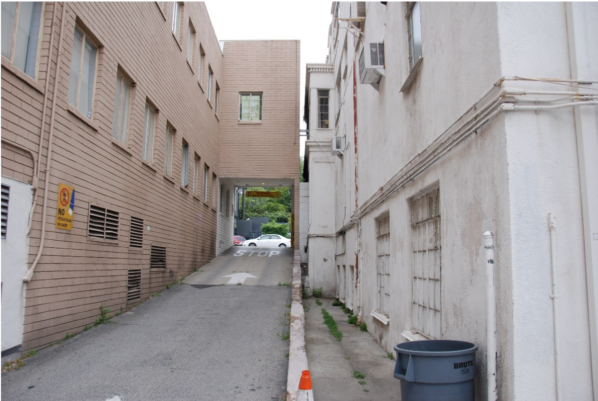
Figure 3b Center of Project Site looking North
