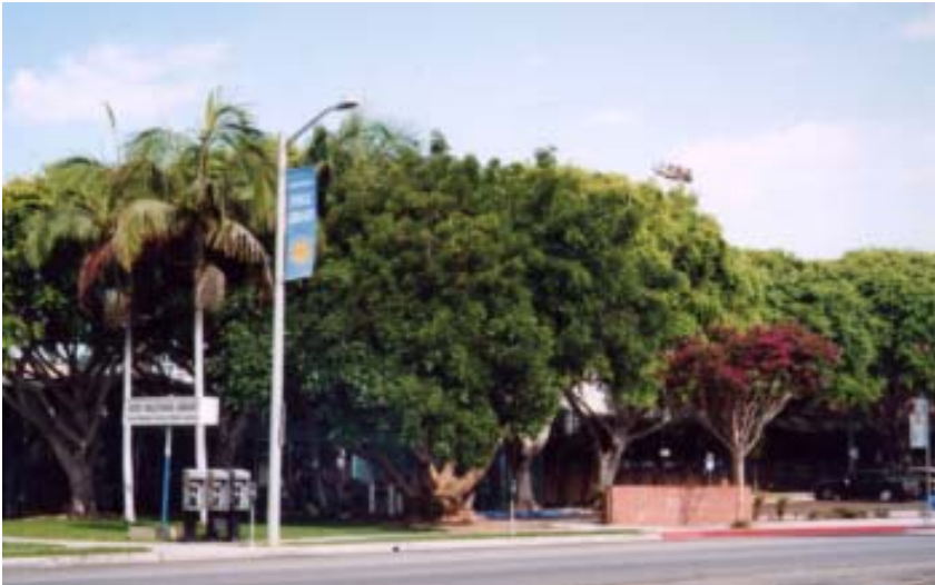
The Library building is set back from the street edge behind a parking lot.
