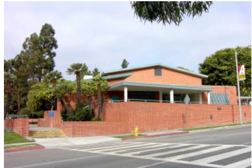
The main pedestrian entrance to the park is a narrow stairway that is not handicap accessible.
