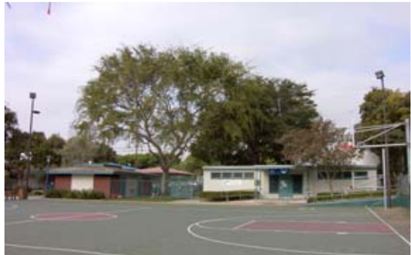
Existing basketball courts are lit with tall high intensity fixtures which is generally acceptable when adjacent to commercial properties.
