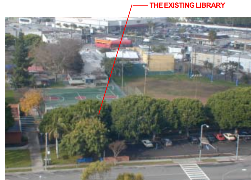
West Hollywood Library. The existing library occupies a site in the middle of the park and faces onto San Vicente Boulevard. Despite the centrality of its location, the library lacks physical presence and visibility from the street and the park.
