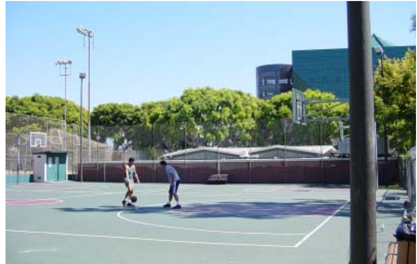
The asphalt paving for the basketball courts creates a large impermeable area that also retains heat.
