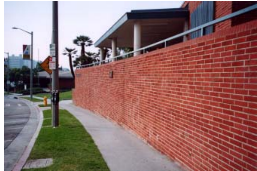
The narrow sidewalk along the Auditorium retaining wall creates a hard edge to the park.
