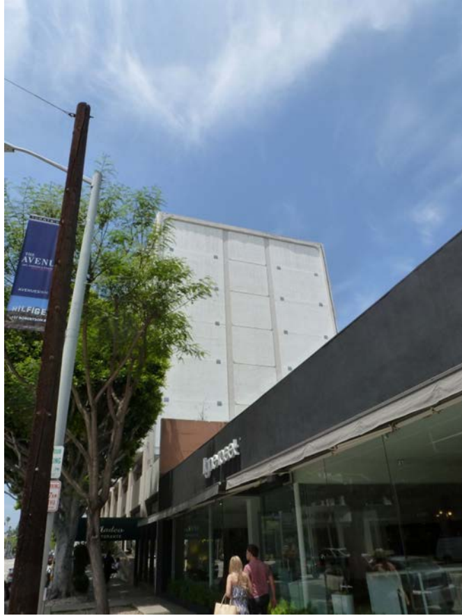
Figure 6: 8899 Beverly Boulevard (1962), east elevation, looking west. Source: GPA.
