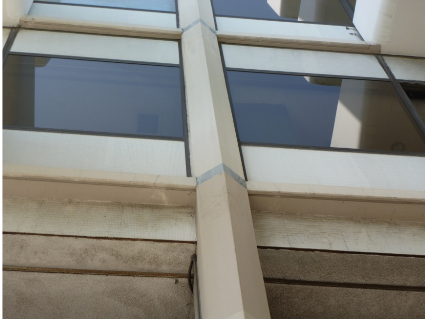
Figure 8: 8899 Beverly Boulevard (1962), north elevation, pier detail. Source: GPA.
