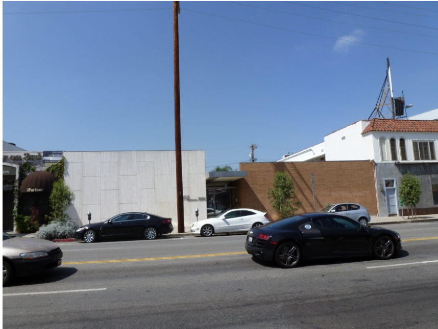
Figure 15: Crescent Professional Building (1959), 8105 W. 3 rd Street, designed by Richard Neutra. Source: GPA.
