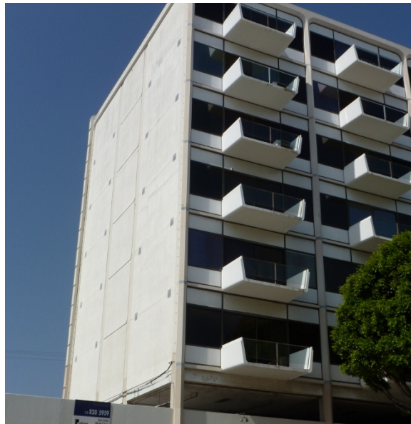
Figure 5: 8899 Beverly Boulevard (1962), west elevation, looking northeast. Source: GPA.
