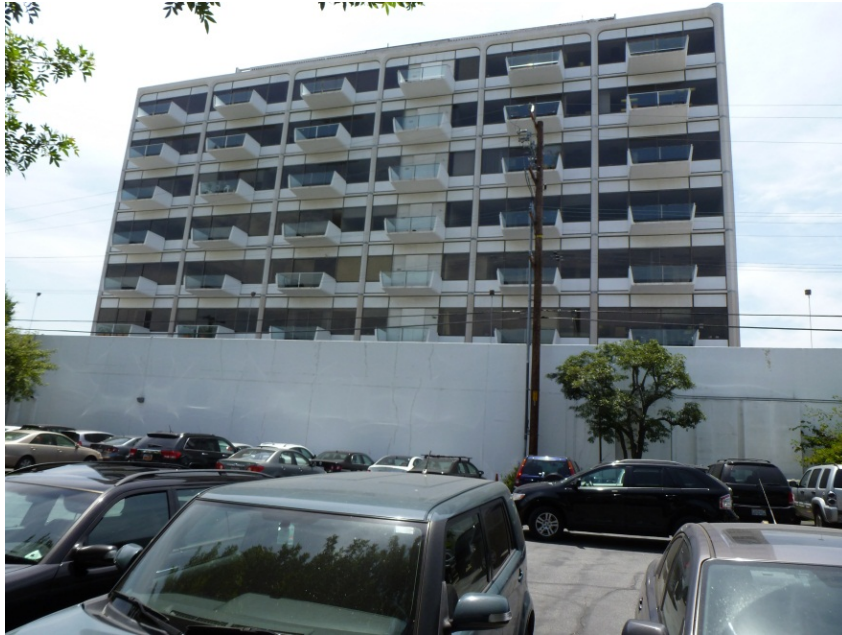
Figure 4: 8899 Beverly Boulevard (1962), north elevation, looking south. Source: GPA.
