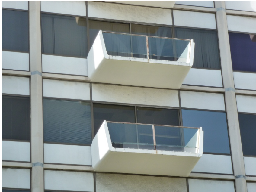
Figure 7: 8899 Beverly Boulevard (1962), north elevation, balcony detail. Source: GPA.
