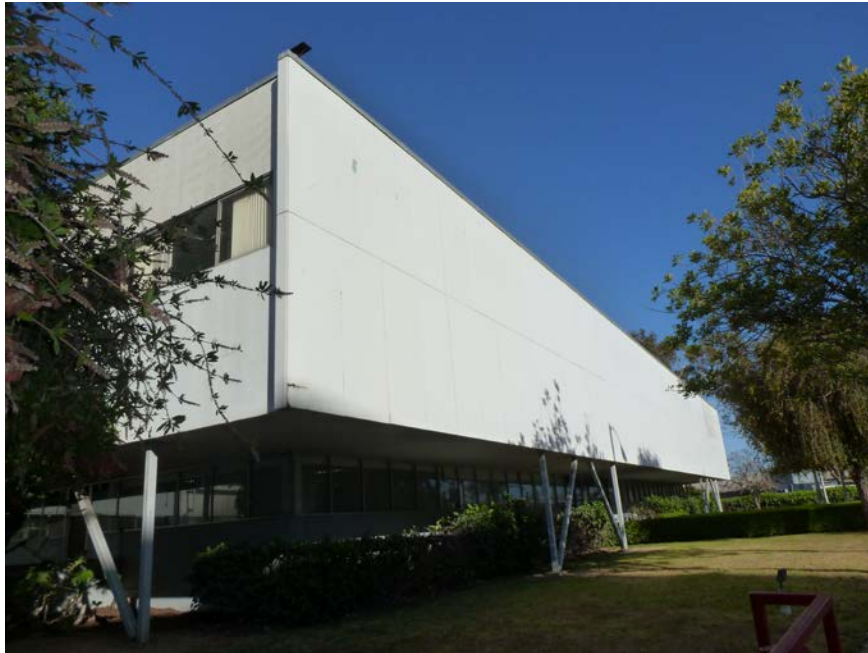
Figure 9: Paper Mate Building (1957), 1681 26 th Street, designed by Richard Dorman. Source: GPA.
